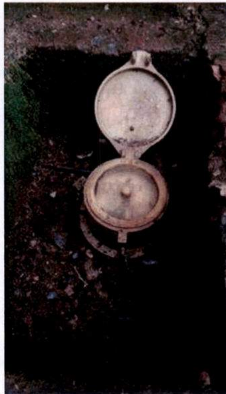
Figure 4-35: Water flow meter installed for RCC OHT
