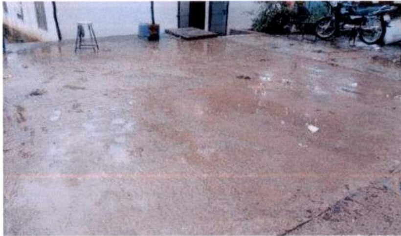
Figure 4-32: Rain water sump at Boy's hostel – 1
