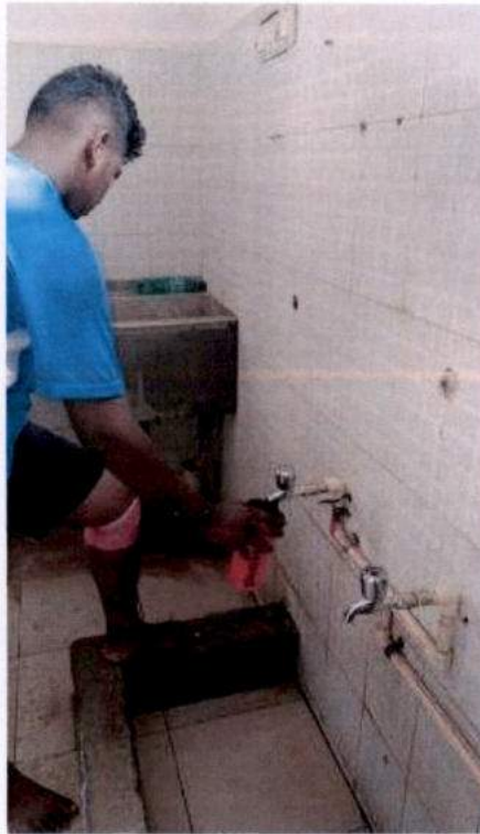
Figure 4-18: RO drinking water consumption point – Boy's hostel
