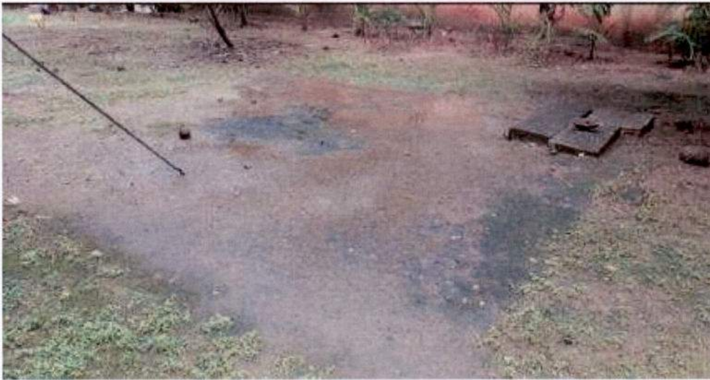
Figure 4-31: Rain water sump at Girl's hostel – 1
