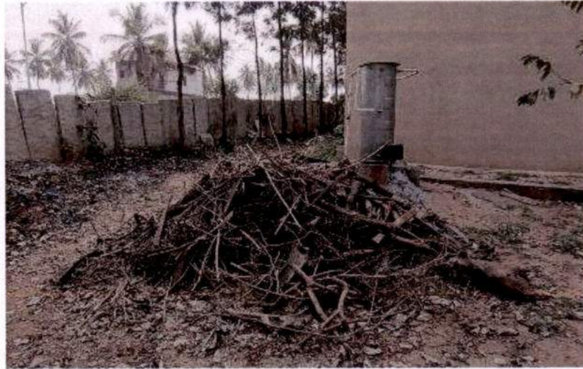
Figure 4-24: Fire-wood boilers for hot water system in Hostels
