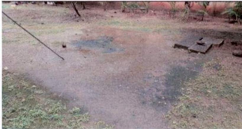
Figure 4-26: Rain water sump at Girl's hostel – 1
