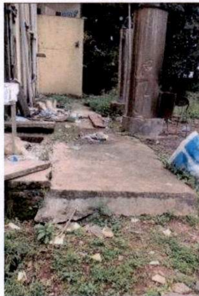
Figure 4-30: Sewage Tank
