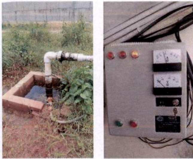
Figure 4-2: Borewell #2 – near Playground (Boy’s hostel side)
