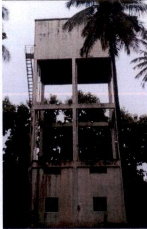
Figure 4-4: RCC OHT – Behind complex block
