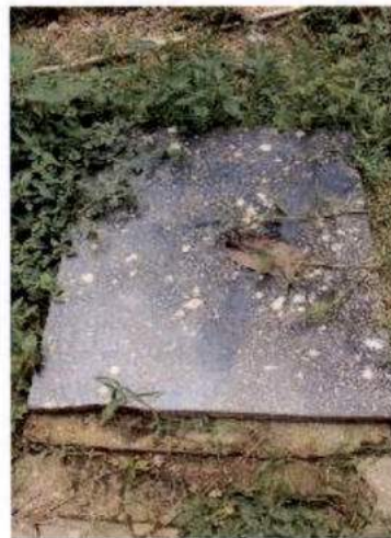
Figure 6-4: Waste Water Chamber
